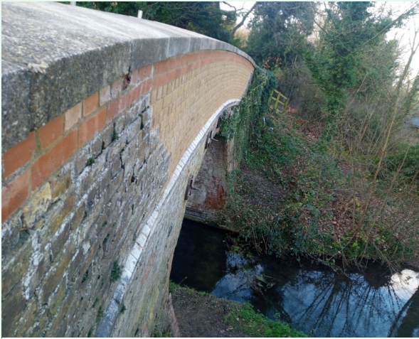
19th December: Repair detail
