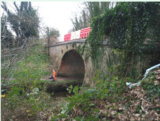
10th December: damaged brickwork removed
