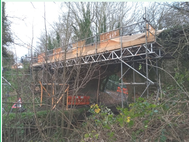
16th December: Scaffolding in place
