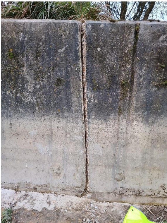
Joint in the bridge hole
