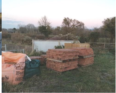
Bricks stored in compound
