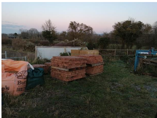
Bricks stored in compound
