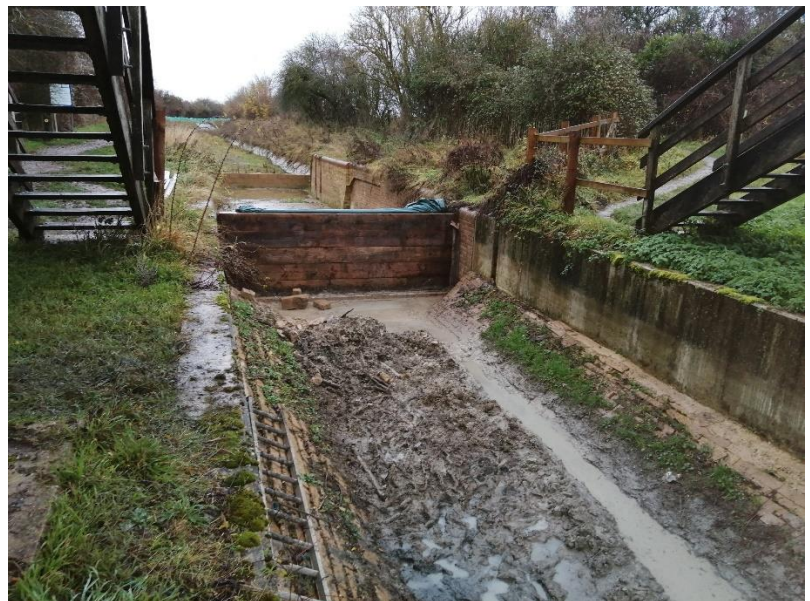
Back of the stop planks with the bed joints exposed.
