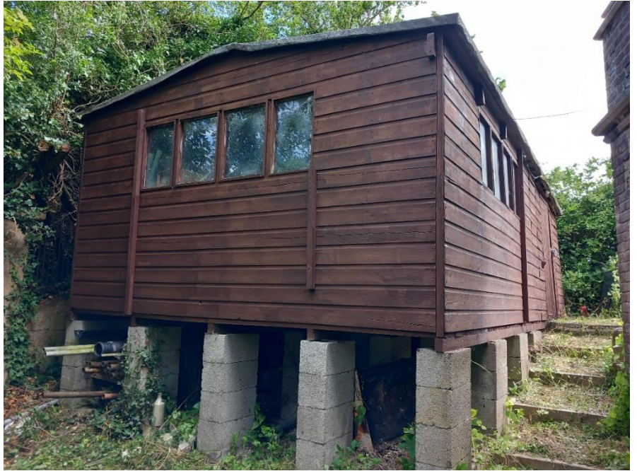
Newly treated timber shed.
