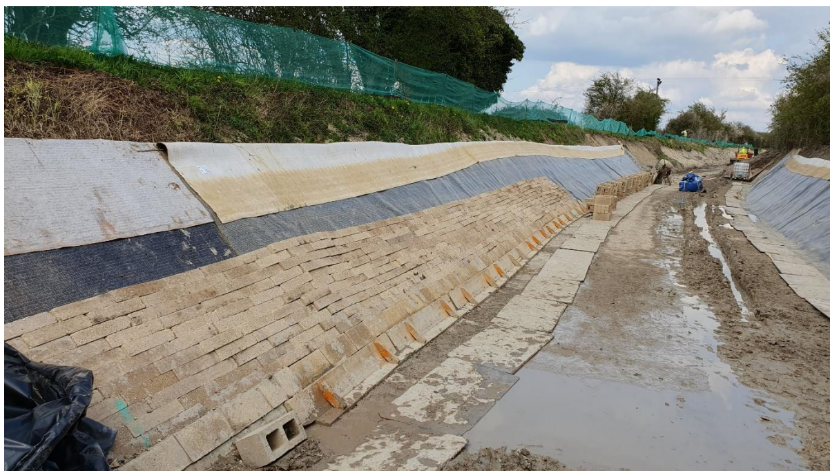
Towpath side with the blocks placed.
