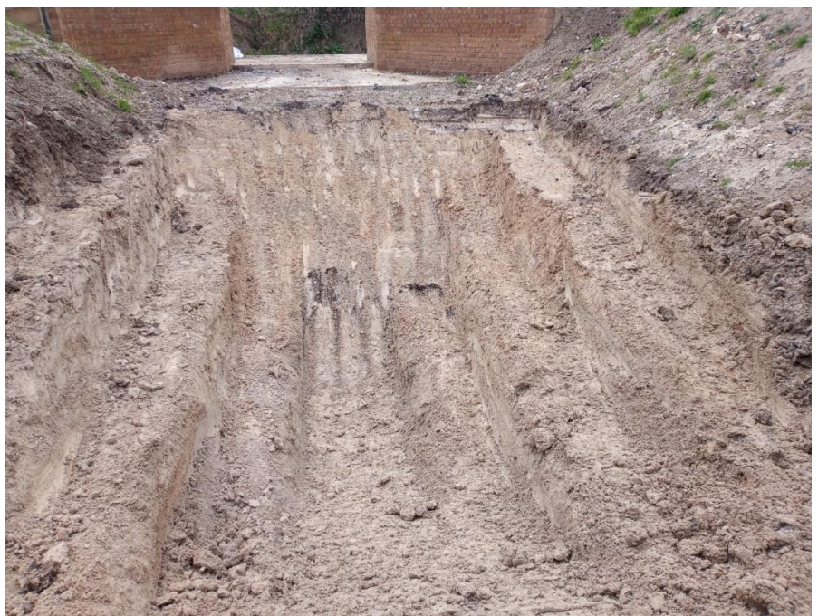
Excavation of terraces below the canal bed.
