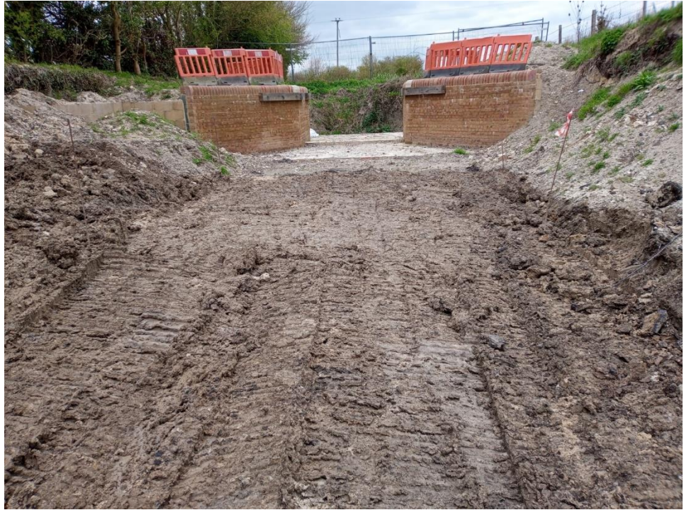
Trial excavation backfilled and compacted.
