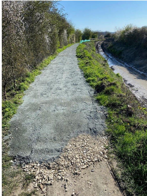
Towpath upgrade complete
