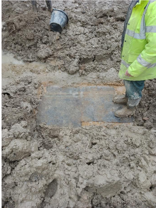
Patch repair to Bentomat.
