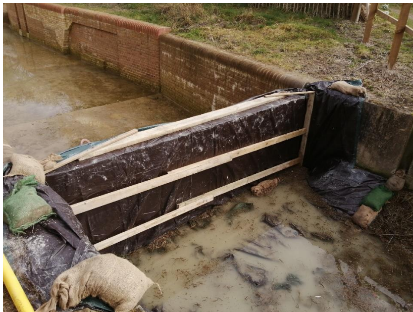
Tarpaulin secured in place.
