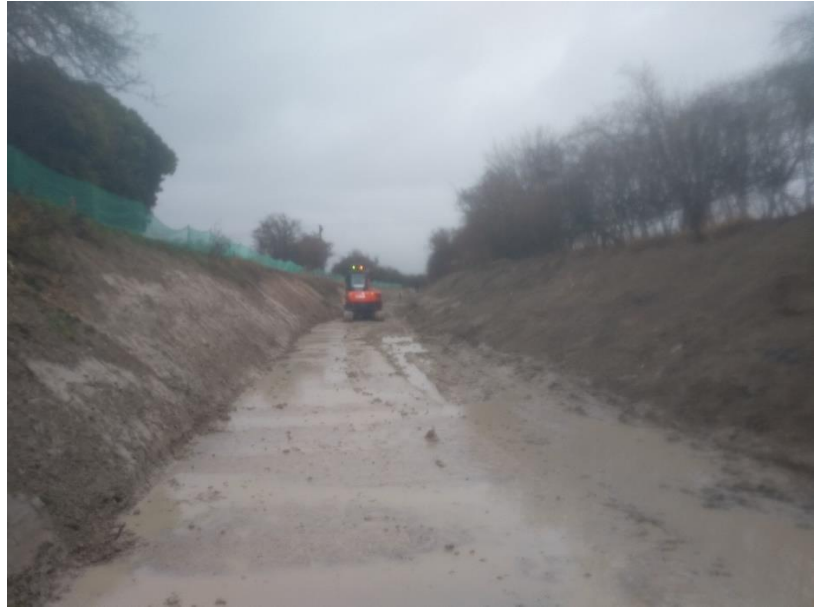
Final profile to the towpath (left) side.
