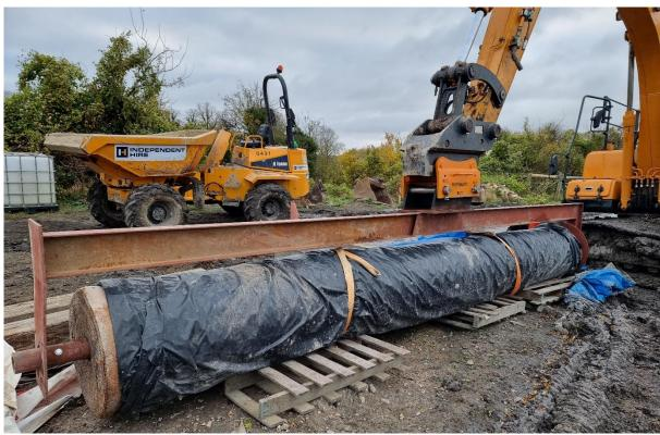
Bentomat dispenser. Note quick-hitch adapter plate and securing bolt under top bracket (on left).
