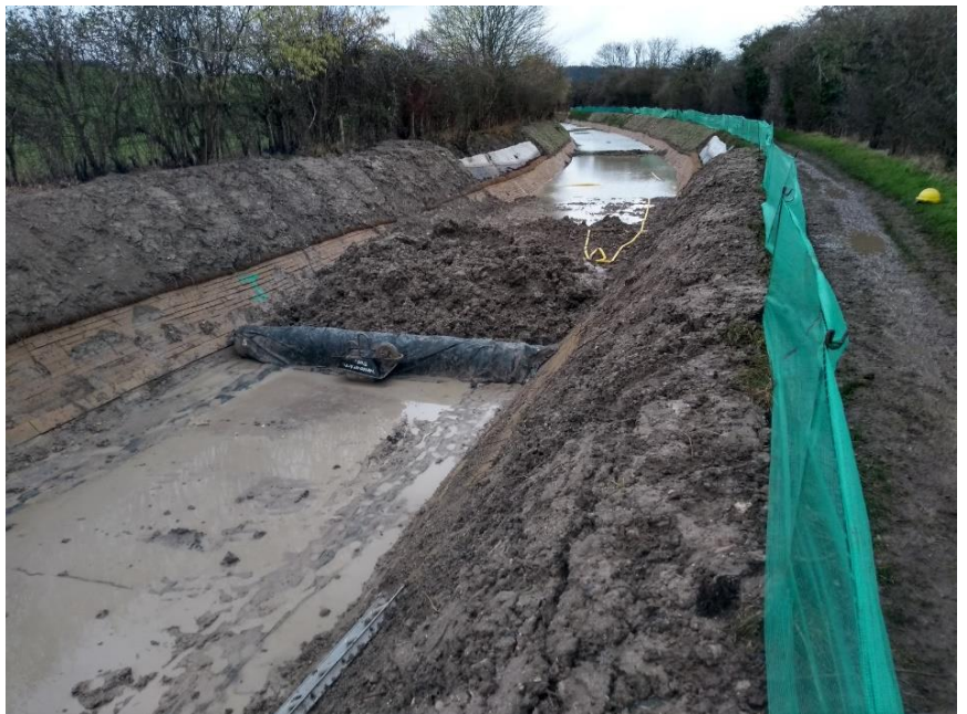
The start of rolling out the bed mat.
