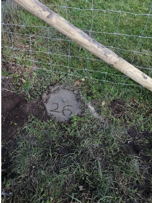
Level control point.
