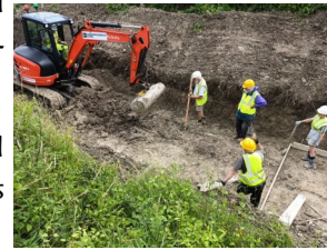
Restoring – slowly but surely... between Bridge 4 and Little Tring
