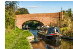
The beautiful, fully restored Little Tring Bridge
