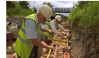
Applying learned skills – building the bank wall near Bridge 4
