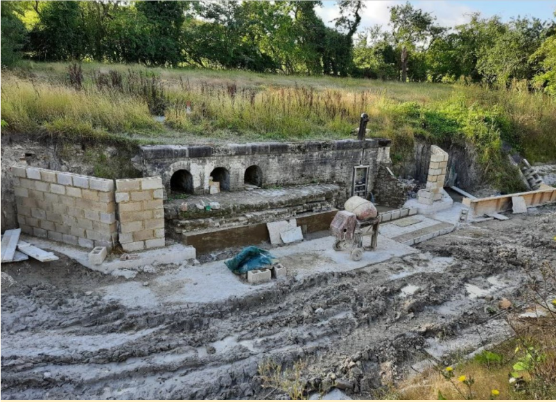
Whitehouses - mid reconstruction
