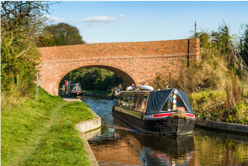
The beautiful, fully restored Little Tring Bridge
