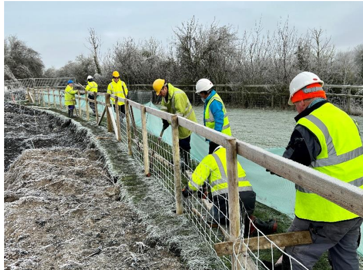
BITM installing the fence on a cold and frosty morning.
