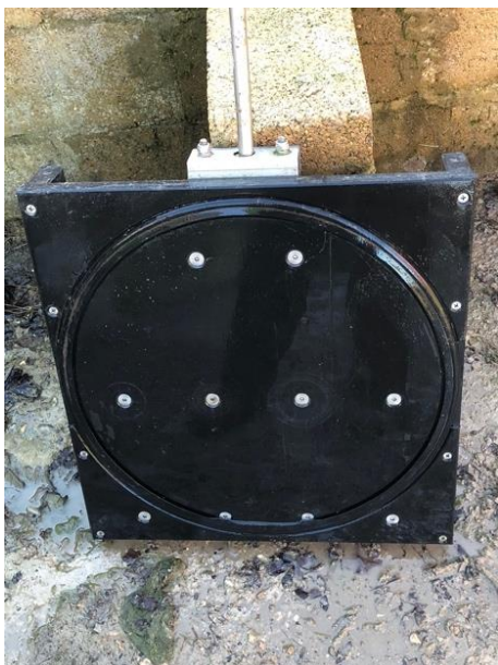
New gasket cut and fitted.
