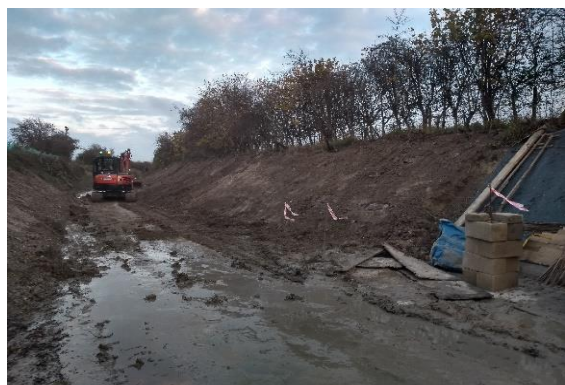
Rough profiling off side bank.
