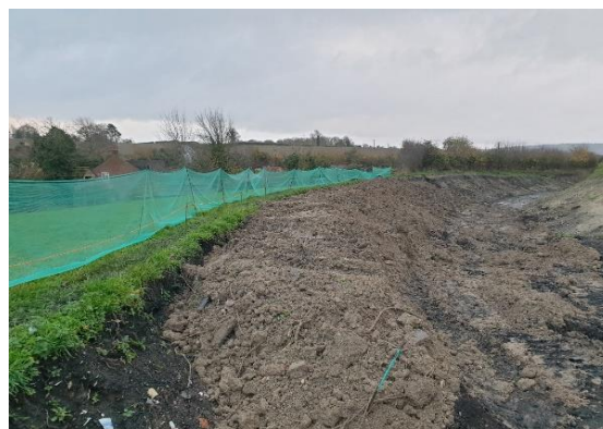
Spoil placed to widen towpath bank.
