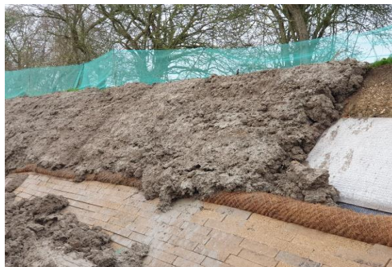
Spoil placed on the towpath bank.
