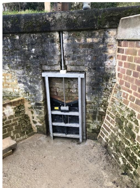
The sluice gate refitted.
