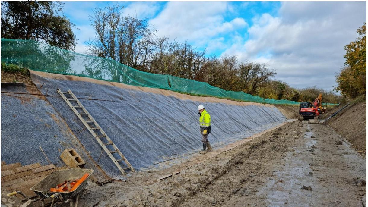
40m Bentomat roll laid. Steel rods & hammering pins home still to be completed.
