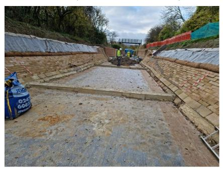
After the" policemen" have cured, spoil is tipped on to the mat at the end nearest the camera and then the spoil is run over by the excavators and dumper to protect the Bentomat and policemen.
