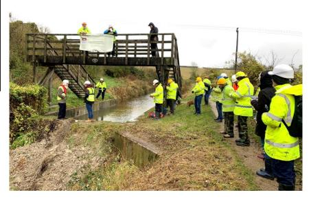
The volunteers standing on the bund with floatation aids are getting ready to lift out the board which is stopping the flow of water from the re watered section beyond bridge 4a. The water in that section is connected to the supply from Wendover so as the level drops it will be replenished.
