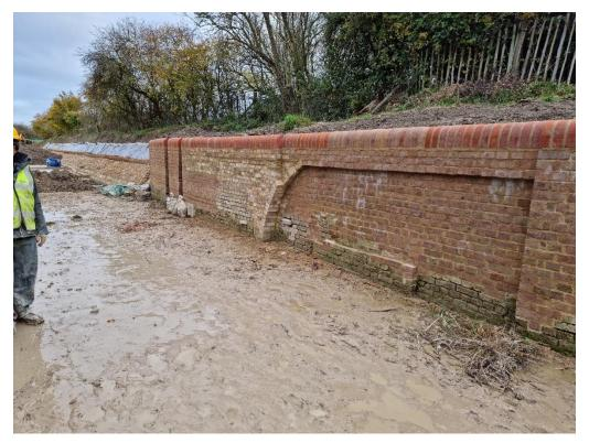
Here we can see the brickwork of Heritage Bricks and Lime mortar virtually complete except for some re-pointing work on the old brickworks lower down. We still don't know what most of the features were for!
