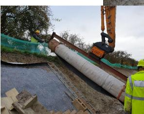
The end of the mat was pinned in position over the existing one and then the mat was rolled out, stopping every metre to put a pin at the top to stop the mat from falling down. We have made a time lapse video of the whole process which can be seen here: - <u>https://youtu.be/7UjCXQfmxuY</u>
