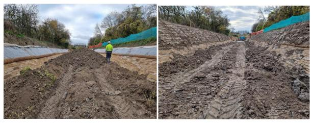
All of the spoil used for back filling contains bits of coal tar from the waterproof lining applied many years ago. This has been separated from "clean spoil which we have found to be possible during the excavation process. The clean spoil is kept separately for disposal. The spoil with coal tar is very expensive to remove but can remain on site.
