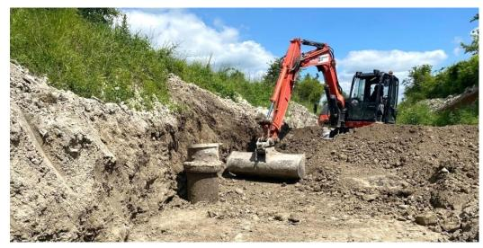
This is the top of the "lamp hole" to enable inspection of the water flow 2m down in the pipeline. To the left is the towpath.
