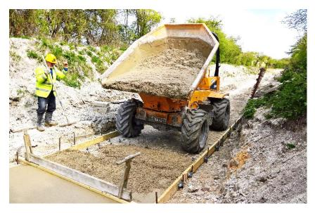
Pipe capping progress has been much improved by placing the concrete "form work" wider apart to allow dumper access. The result is also a wider "road" that will be used for subsequent excavation and lining work thus avoiding the churned mud we usually suffer from in winter.
