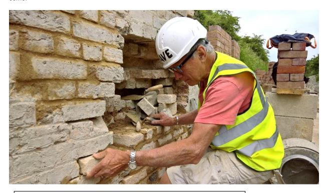
The Old Swing Bridge walls are meticulously repaired with heritage bricks and lime mortar after the loose bricks and old mortar have been removed
