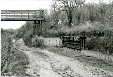
Shuttering ready for concrete pour at bridge 4 — bring on the warmer weather!
