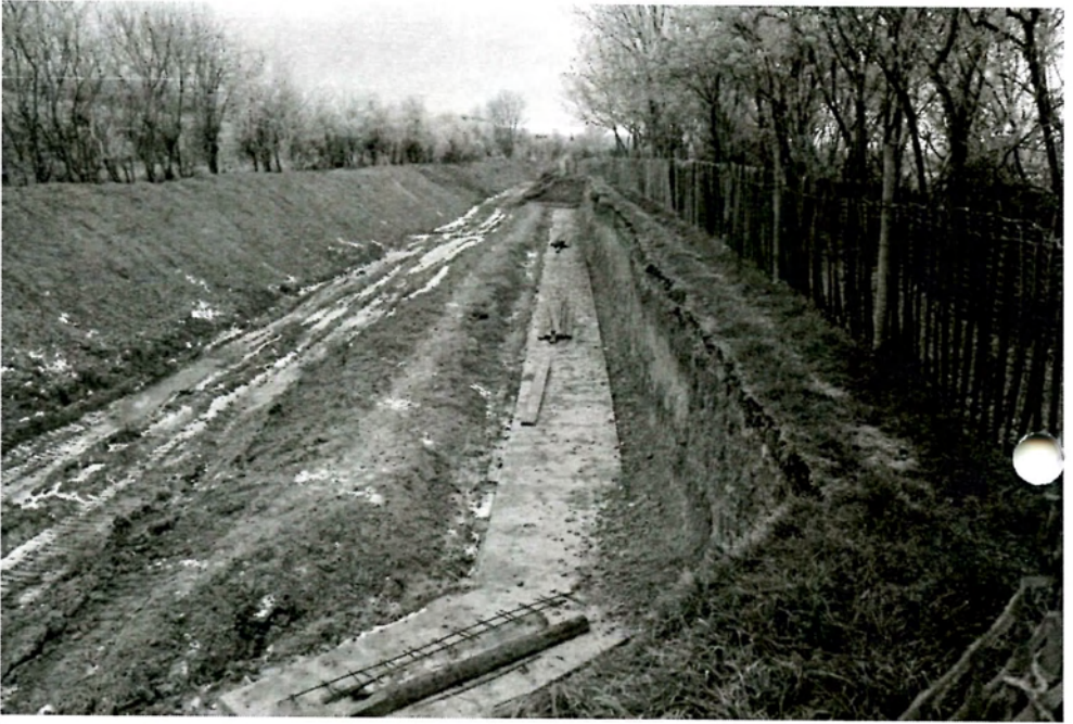
Blinding cast at second mooring bay
