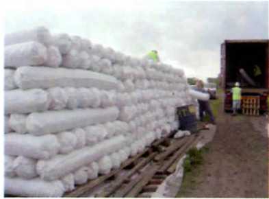
Rolls unloaded and stacked
