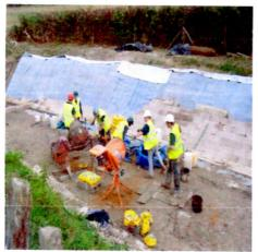
it with a bentonite clay material that keeps the canal watertight. The sloping sides that will be under water have to be covered with concrete blocks to protect the clay lining.
