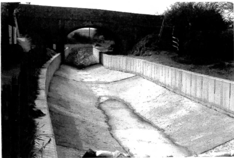
Phase 1 Progress: the completed lining has advanced under Little Tring Bridge, and should have extended further still by the time this magazine appears.
