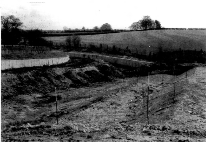
Phase 1 Progress: the winding hole takes shape. The offside bank in the foreground will have a soft edge, planted with aquatic vegetation.
