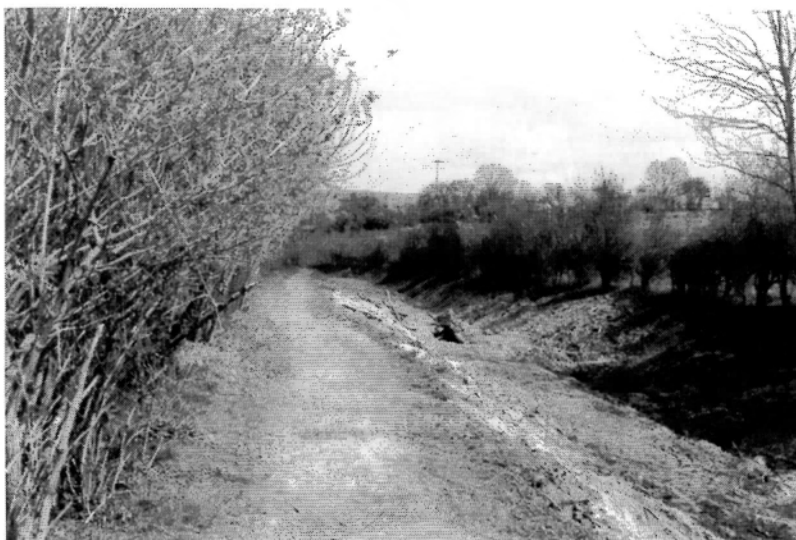
Phase 2 Progress: there it was, gone! After all those years of 'scrub bashing', breakthrough has occurred and the 1¼ mile dry section is now clear (apart from the odd large stump) and re-profiled ready for lining.
