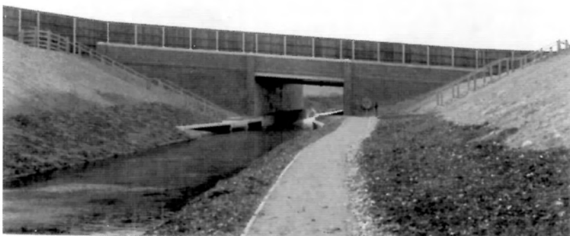
The new A41 road bridge, viewed from the Drayton Beauchamp side. Since the road opened, a substantial wooden fence has been built on this side, and can be clearly seen in this picture. It is very effective at deflecting traffic noise, and the canal on this side of the road is remarkably quiet.
