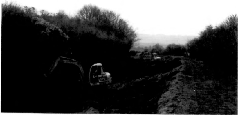
Following the scrub clearance the excavators (crewed by Ray Orth and Ron Pittaway) profile the bed ready for lining.
