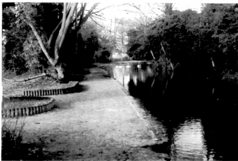
Part of the improved towpath at Wendover Basin.
