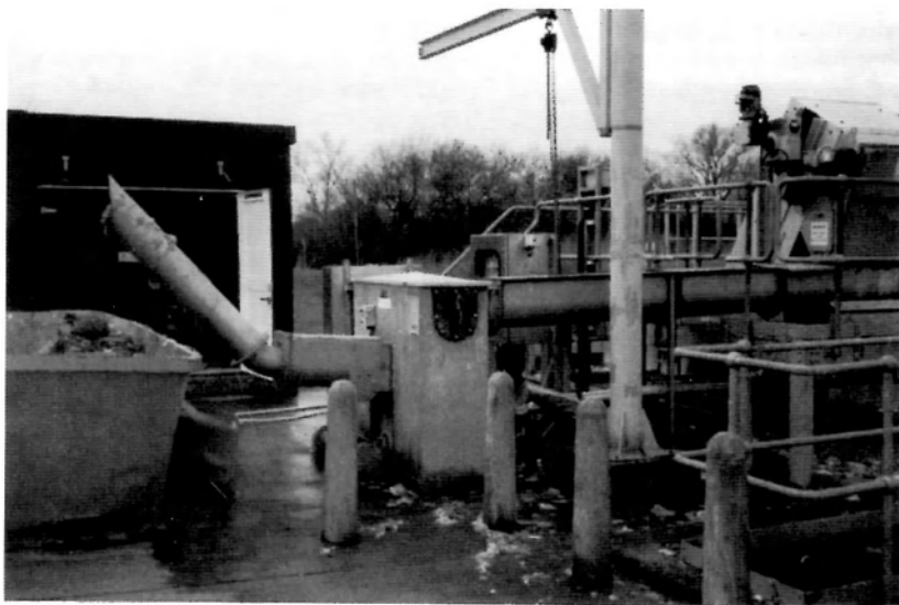
The smelly bit! Rags, extracted by the filter and lifted by the device on the right, are deposited in a skip (after the 'juice' has been squeezed out).
