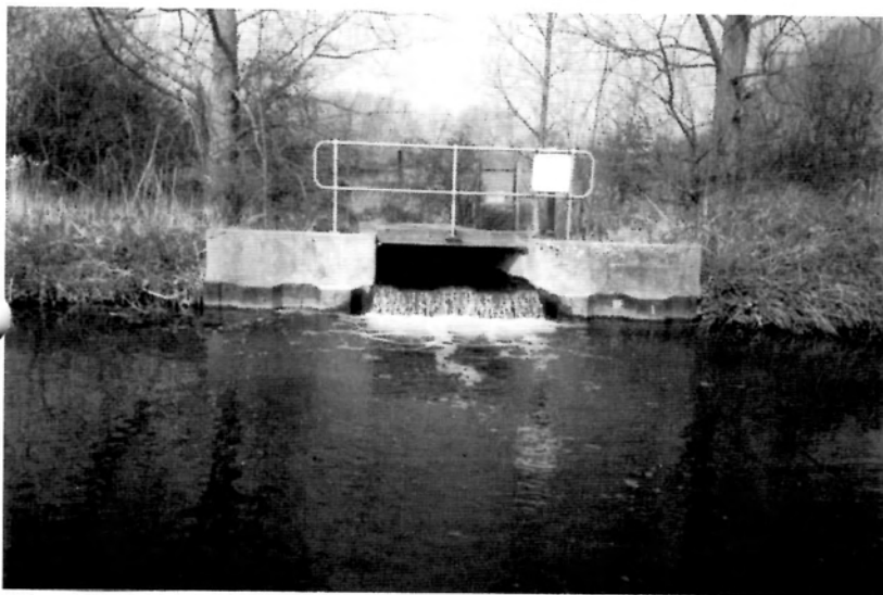
The treated effluent, an average of 220,000 gallons a day, is pumped into the Arm at the familiar outfall near Gamnel Bridge.
