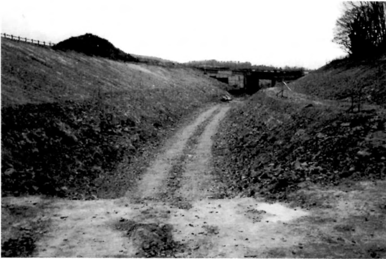
Looking west towards the new road bridge, as yet without brick facing. The depth of the new canal cutting can be appreciated from the ground level, which is at the fence on the left and trees on the right. The original canal is beyond the trees. This section will be lined by Balfour Beatty in the Spring, when ground conditions improve.
