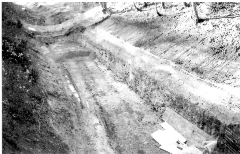
The view looking west from Drayton Bridge showing the excavated channel prior to lining. The pipeline ran to the left of the channel and the exposed pipe can just be seen towards the top left of the picture.
