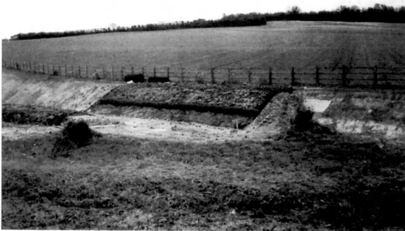
This is the trial section of lining, near where the new canal diversion meets the original line west of the by-pass (very weedy bit of original canal just discernable in the foreground). Note the coir roll at water level. The Bentomat has been covered with spoil.
