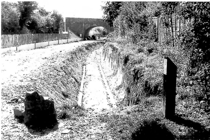
Looking from the stop lock along the newly excavated towpath side trench after demolition of the old wall and prepared ready for construction of the new wall. The re-instated public footpath is behind the paling fence on the left.
