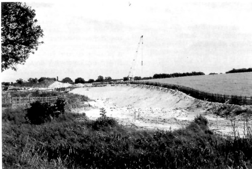
A view from the point where the new canal joins the old line, west of the new A41 road crossing, showing the recently excavated cutting which will take the new section of canal.
