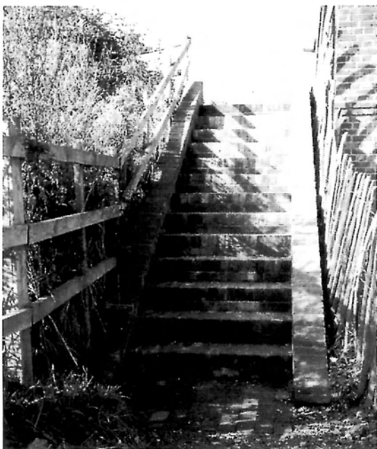
The final part of the Little Tring Bridge Contract was to build steps for the public footpath from the road to canal level. These smart new brick steps were installed by Priory Construction during July.
