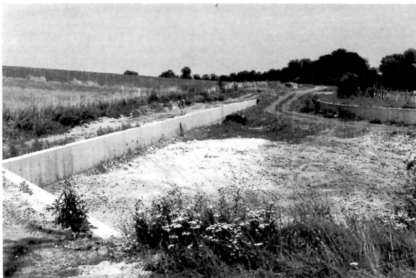
The newly excavated winding hole at Little Tring, showing completed walls.
