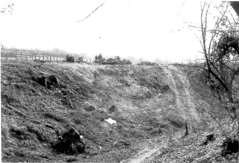
This is the point at Drayton Beauchamp where the new line diverges from the existing (looking south west). The cleared bank opposite will be excavated to create a cutting. There will be a public footpath along the new towpath from this point, and the existing public footpath along the old towpath will be retained as far as the present sump.
