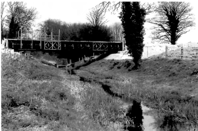
This view shows the present sump, looking east. The bridge is a temporary Bailey structure to provide a crossing for the contractors; the new road will cross the old canal line on an embankment at this point. The section of canal in the foreground will become the reed bed for processing the road run-off.
