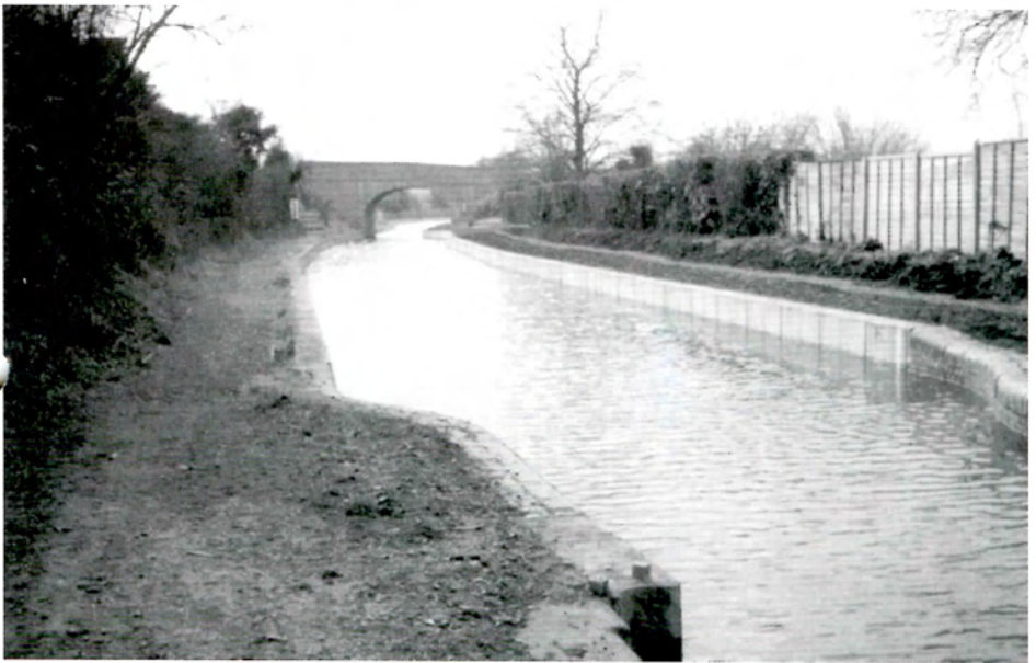
Almost full, about 6" off. Compare this shot with the one on the front cover of the previous 'Wendover Arm News', taken in 2000, as it is taken from the same spot.
