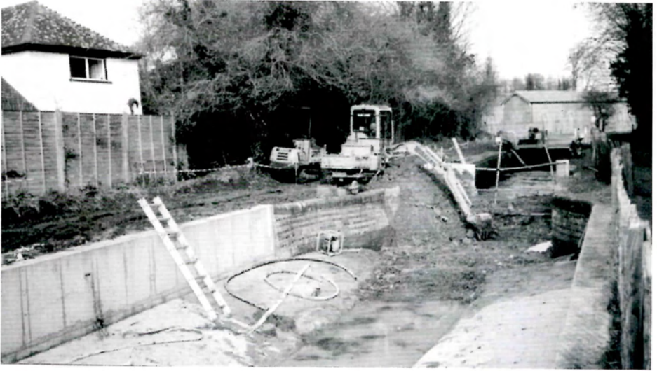
Above: removing the bund, prior to re-watering on 6th March 2005.
