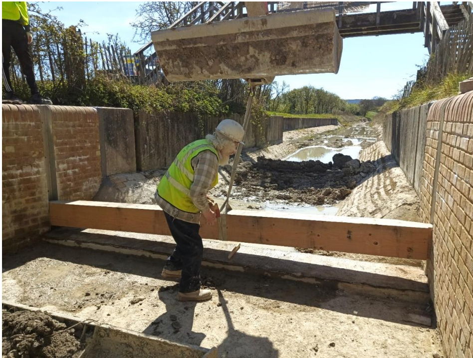
Here is the first plank being put into position
