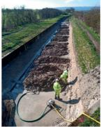
place to pump out the rainwater. The work area was pumped out quickly, so the opportunity was taken to pump out the large lake just before the work area and the semi-finished bed and concrete policemen on the other side of bridge 4
