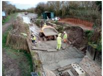
The whole of the concrete mass was deaerated with a vibrating poker. This tended to allow the wooden form work to float up and some time was spent putting in more pins in strategic positions to show what the concrete level needed to be.
