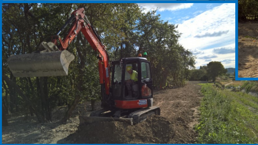
Final levelling of the track on the offside area near Whitehouses.
