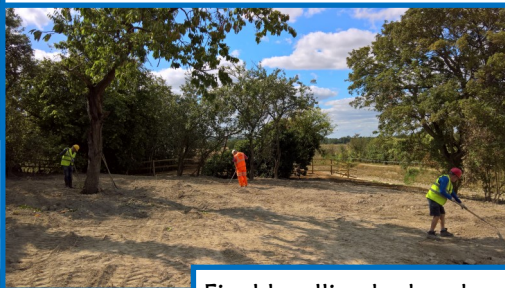
Final levelling by hand using rakes prior to seeding at the Whitehouses site.
