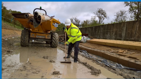
Offside bank work linking the lining to the mooring wall.
