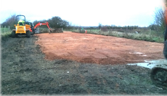
(left) MOT type I was added and rolled to make the rough places plane and . . .
