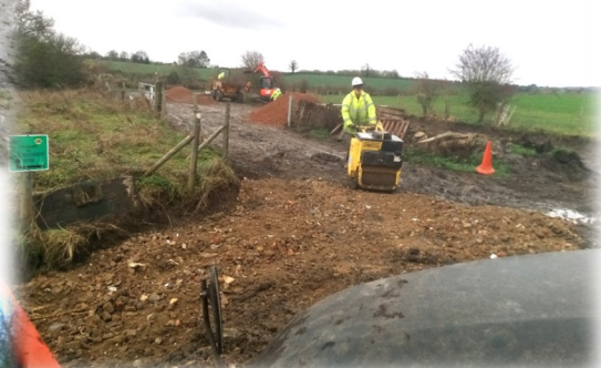
(above) And the mud was separated from the land with crushed concrete and . . .
