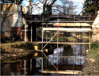
railings removed and scaffolding in place
