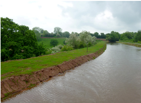
The repaired breach at Halberton
