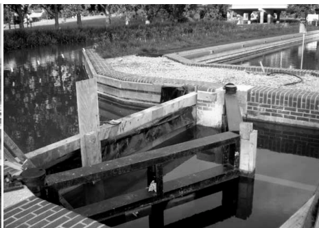
The stop-lock, waiting for the bridge to be emplaced
