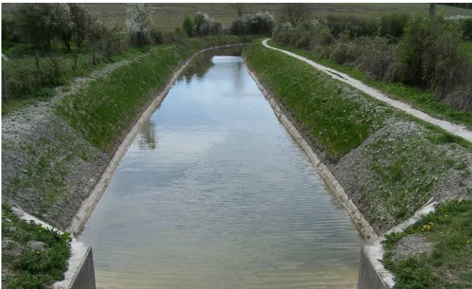
RE-WATERING NOW REACHES BRIDGE 4A
