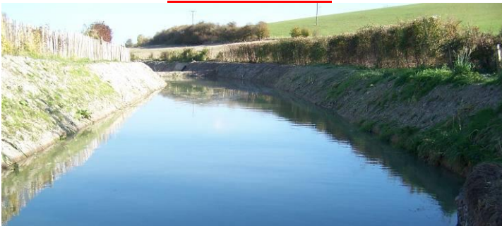
60 METRE TEST SECTION IN WATER AT DRAYTON BEAUCHAMP
