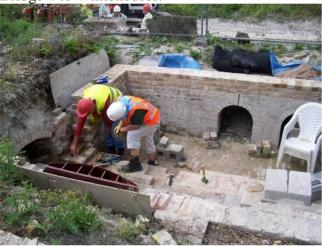
KESCRG RESTORING THE WALLS OF THE OLD SETTLING TANK WITH WEIR THAT IS GOING TO BE BROUGHT BACK INTO USE AFTER RE-WATERING
