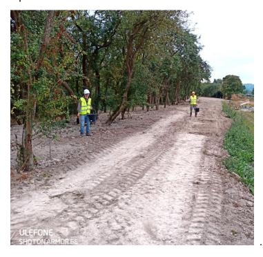
All the topsoil was finally distributed and raked by hand before grass seed was sowed.
