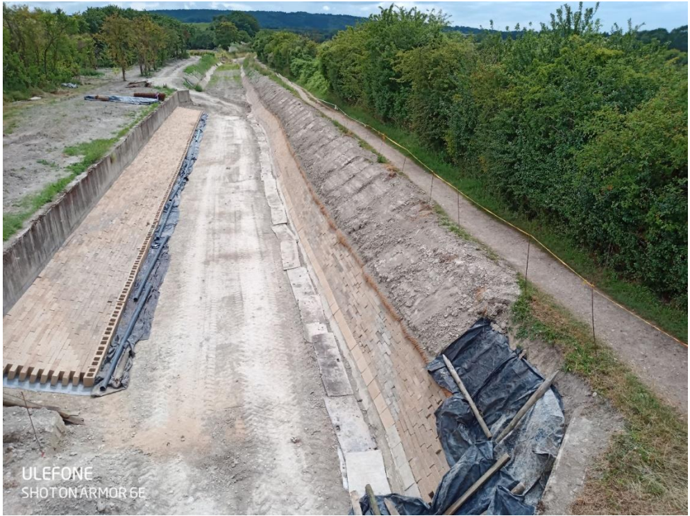
Left - View from top of bridge 4
