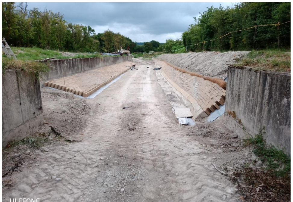
View under bridge 4
