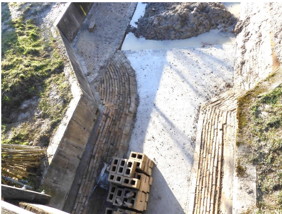
The view looking directly down from bridge 4
