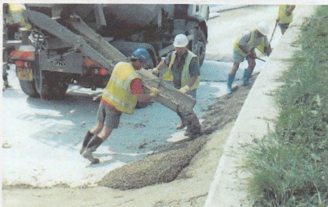
POURING SOME OF THE 470 TONNES OF READYMIX
