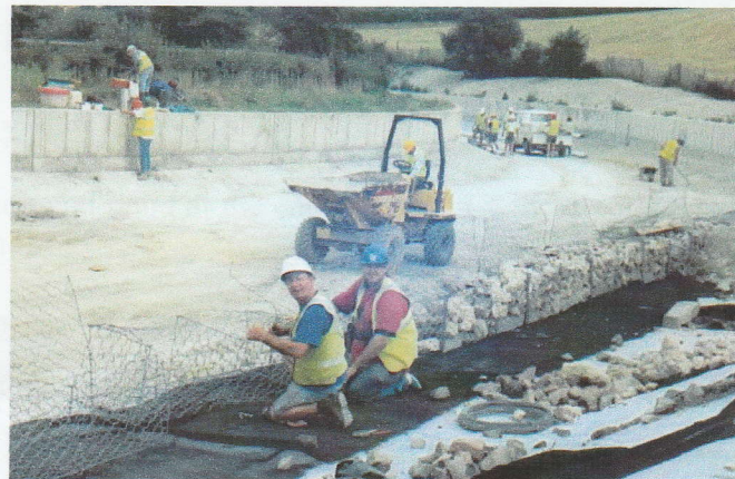
DRY STONE WALLERS HARD AT WORK ON FILLING THE GABIONS
