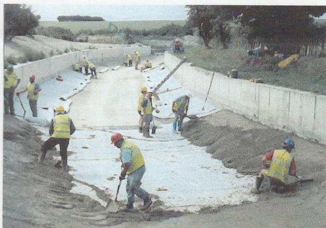
BY TUESDAY THE CONCRETING WAS WELL AWAY FROM THE BRIDGE AND THE BENTOMAT LAYING TEAM WERE NEARING THE WINDING HOLE
