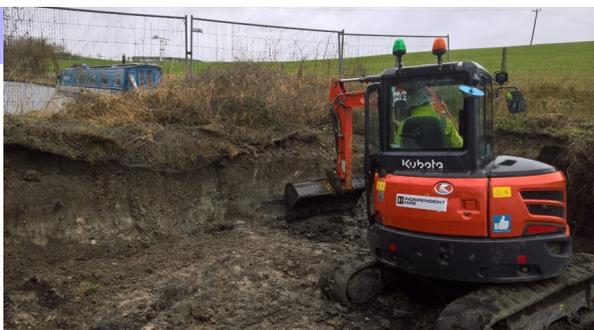
boats trying to go any further, since they would not be able to pass any other boat as they go through our relined channel. We have been carefully excavating next to the winding hole, to expose the end of the Phase 1 concrete walls and lining. Pictures by Steve Bonser.
