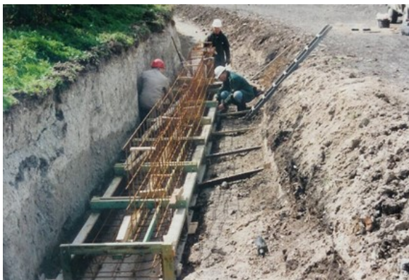
The base formwork being prepared for the first 8.8m pour in April 1999
