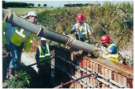
Ready-mix being poured into a wall
