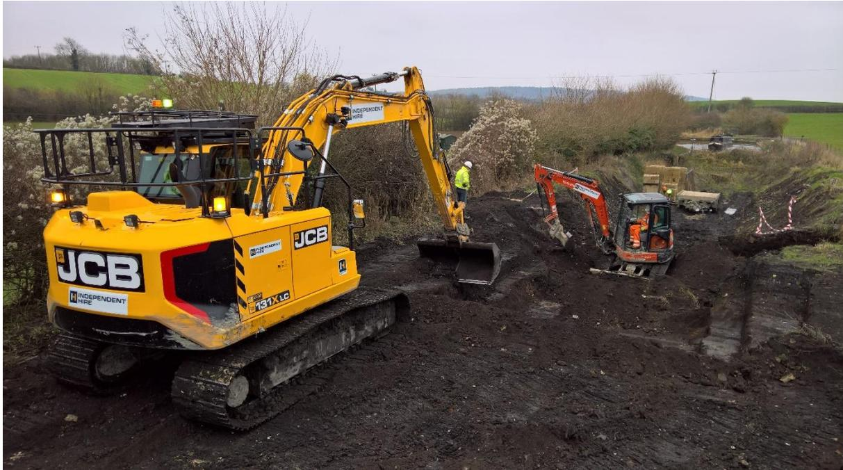
The above picture shows ash being dug out. In the background is a narrow boat “winding” (turning) at the current head of navigation (which we opened in 2005). The ash is about to be loaded into a dumper and taken to the pile shown on the previous page for removal. At the end of the working party, all the ash previously piled up at this location near the winding hole had gone, and most of the ash on which that pile was standing, has also been dug out.
